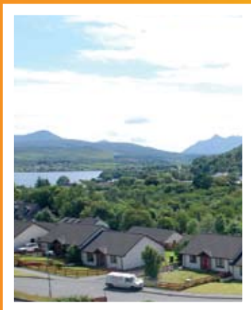
The foundations for future regulation
